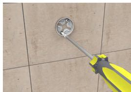
2. Align flexi-fix wall plate to existing fixing points rotating as necessary. Fix in place using the screws provided.
